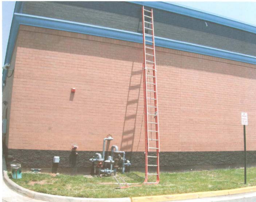
Ladder collapsed – worker was able to grab on to the leading edge of the building
