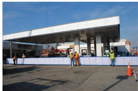
Contractors use barricading walls and/or fencing for larger projects
