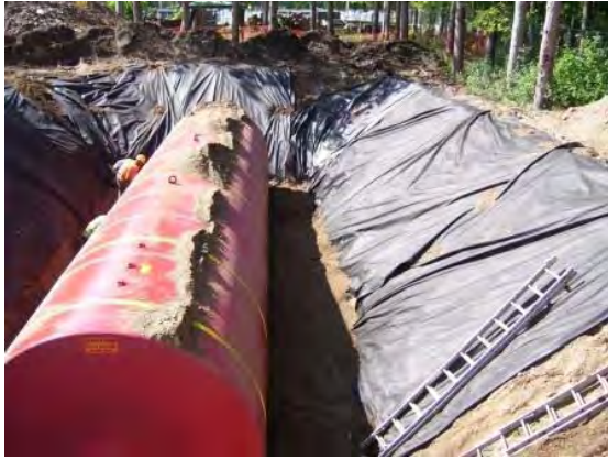
Tamping and compacting the first lift
